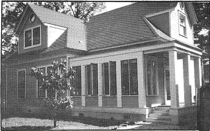
THE MARBLE HOUSE, C. 1908 4112 Avenue F
