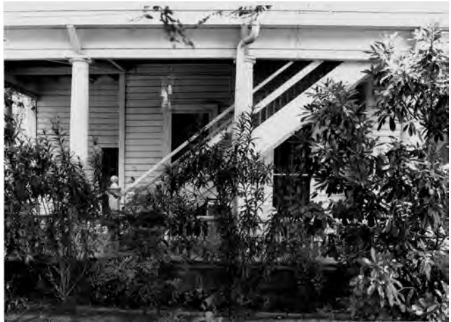
FRONT PORCH STAIRCASE
