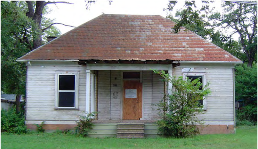
SCHENKEN-OATMAN HOUSE PRE-RESTORATION, AFTER REMOVAL OF METAL SIDING
