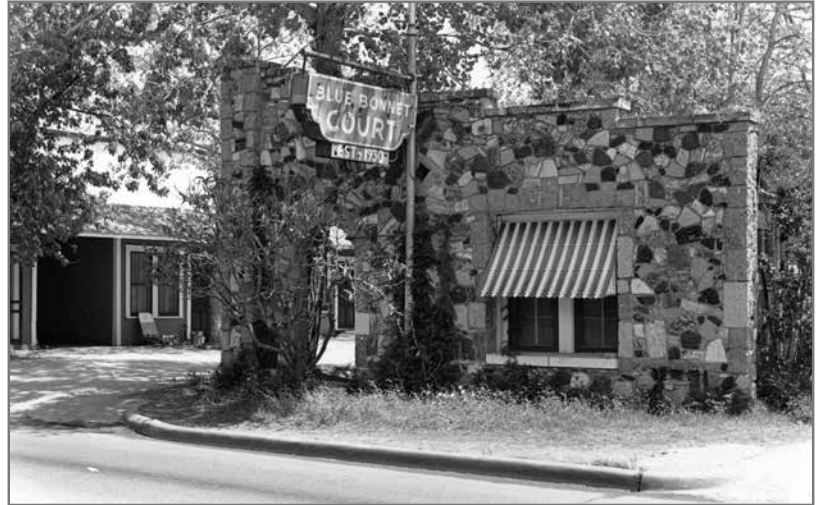
A photo of Blue Bonnet Court included with the property's application for entry in the National Register of Historic Places, presumably taken around the same time of the application in 1990. Image: National Register of Historic Places
