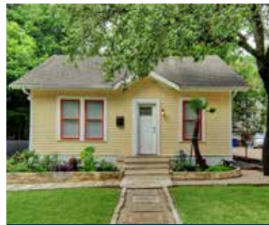
605 East 43rd Street
