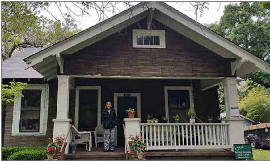
Joan in Front of Her House in Progress, with the Asphalt Covering Revealed
