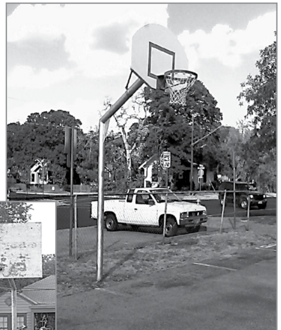
Baker Center backboard & hoop installation, before (left) - by Karen McGraw and after (above) - by Paul Kamprath
